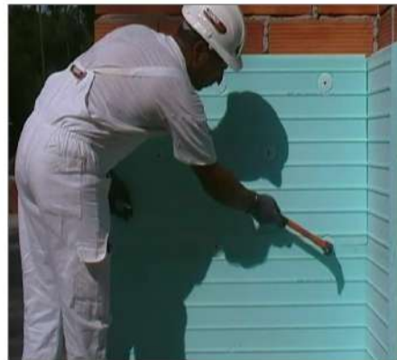
Hammer the fasteners
