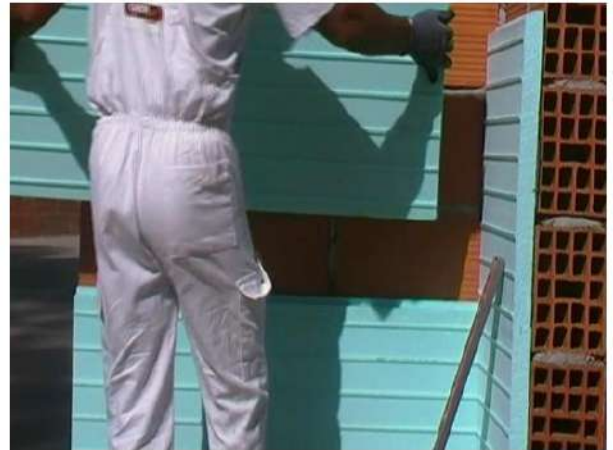
Placing the board in the substrate
