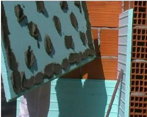
Placing the adhesive on the board
