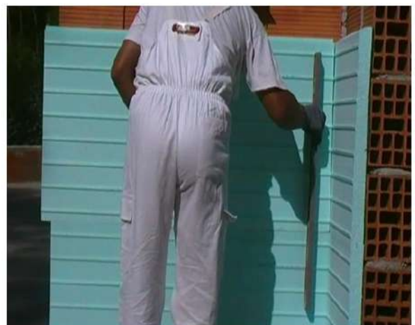
Leveling the boards
