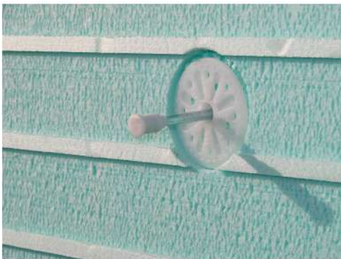
Placing the fasteners
