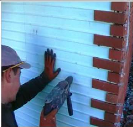
Drilling with 10mm thickness
